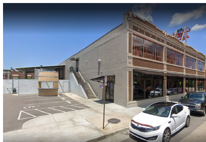
Low Impact Industrial Use : Microdistillery on South Front St
