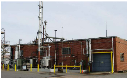
Manufacturing Facility on Chelsea Ave
