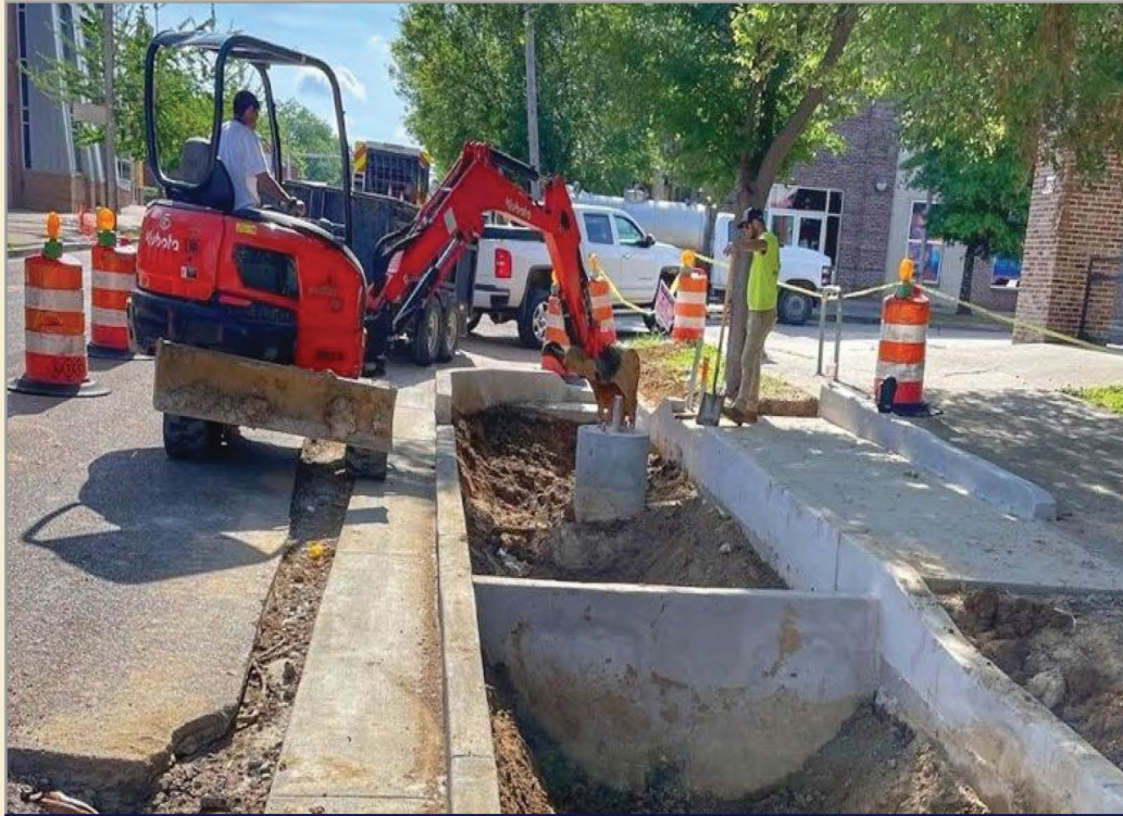
MCLEMORE AVENUE GREEN INFRASTRUCTURE (BIOSWALE)
