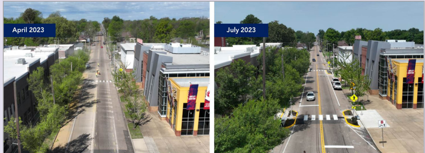
EARLY STAGE INVESTMENT (ESI) ON MCLEMORE AVE INCLUDED THE INSTALLATION OF TWO MID-BLOCK PEDESTRIAN CROSSINGS, RECTANGULAR RAPID FLASH BEACONS (RRFB), AND THE CITY'S FIRST INSTALLATION OF GREEN INFRASTRUCTURE CALLED BIOSWALES. PROJECT COMPLETED IN JULY 2023. PHOTO LOOKING WEST ON MCLEMORE AVE.
